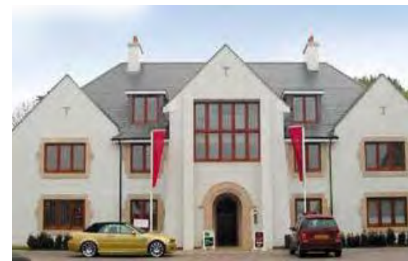
New build examples of the ongoing appeal of an Arts and Crafts aesthetic can be found in Guildford
