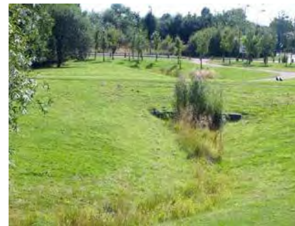
Where attenuation areas are mainly dry, other than in storm events, they can be used as open space.
