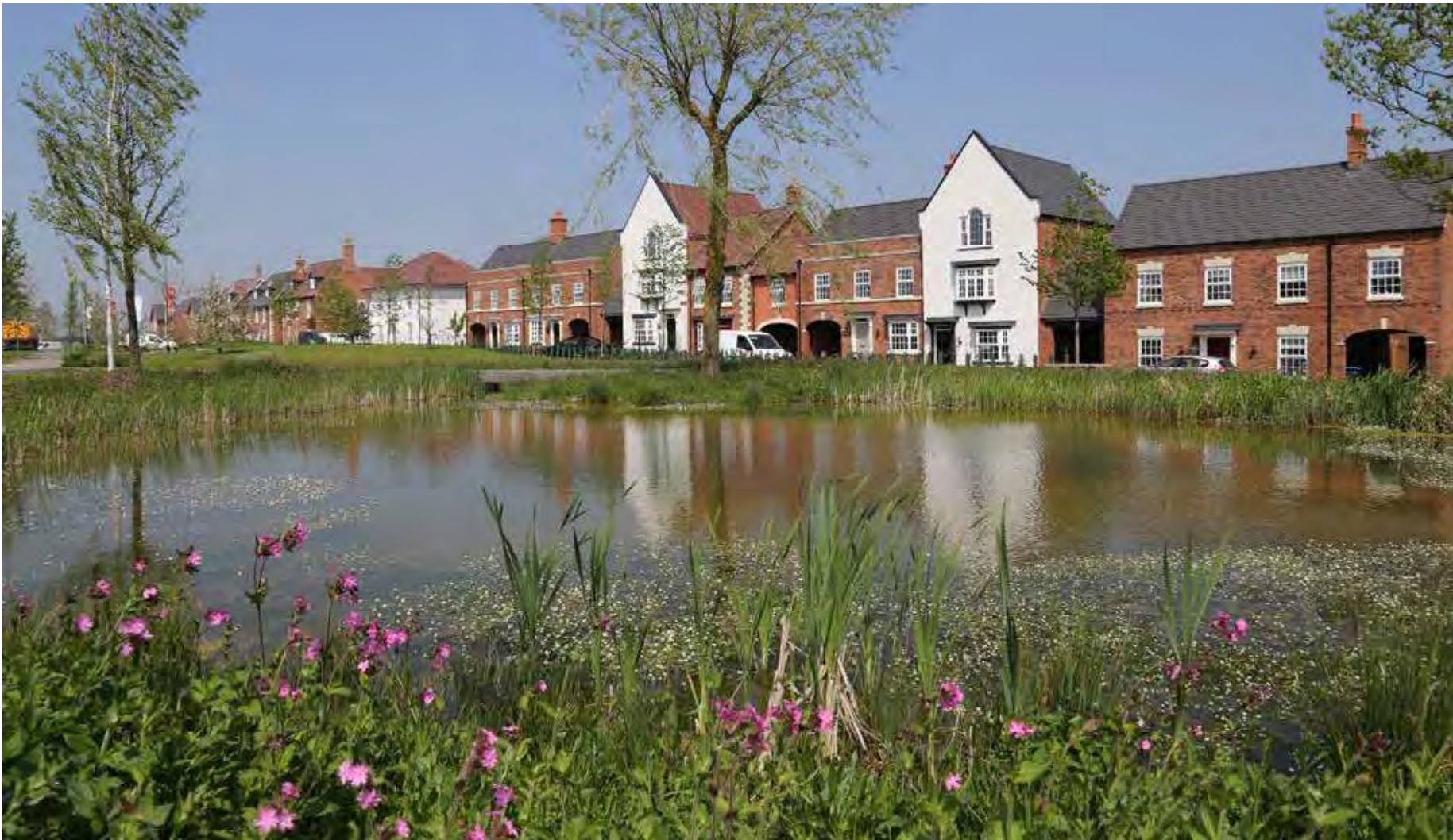
SuDS can add an attractive amenity asset to new residents whilst providing biodiversity benefits
